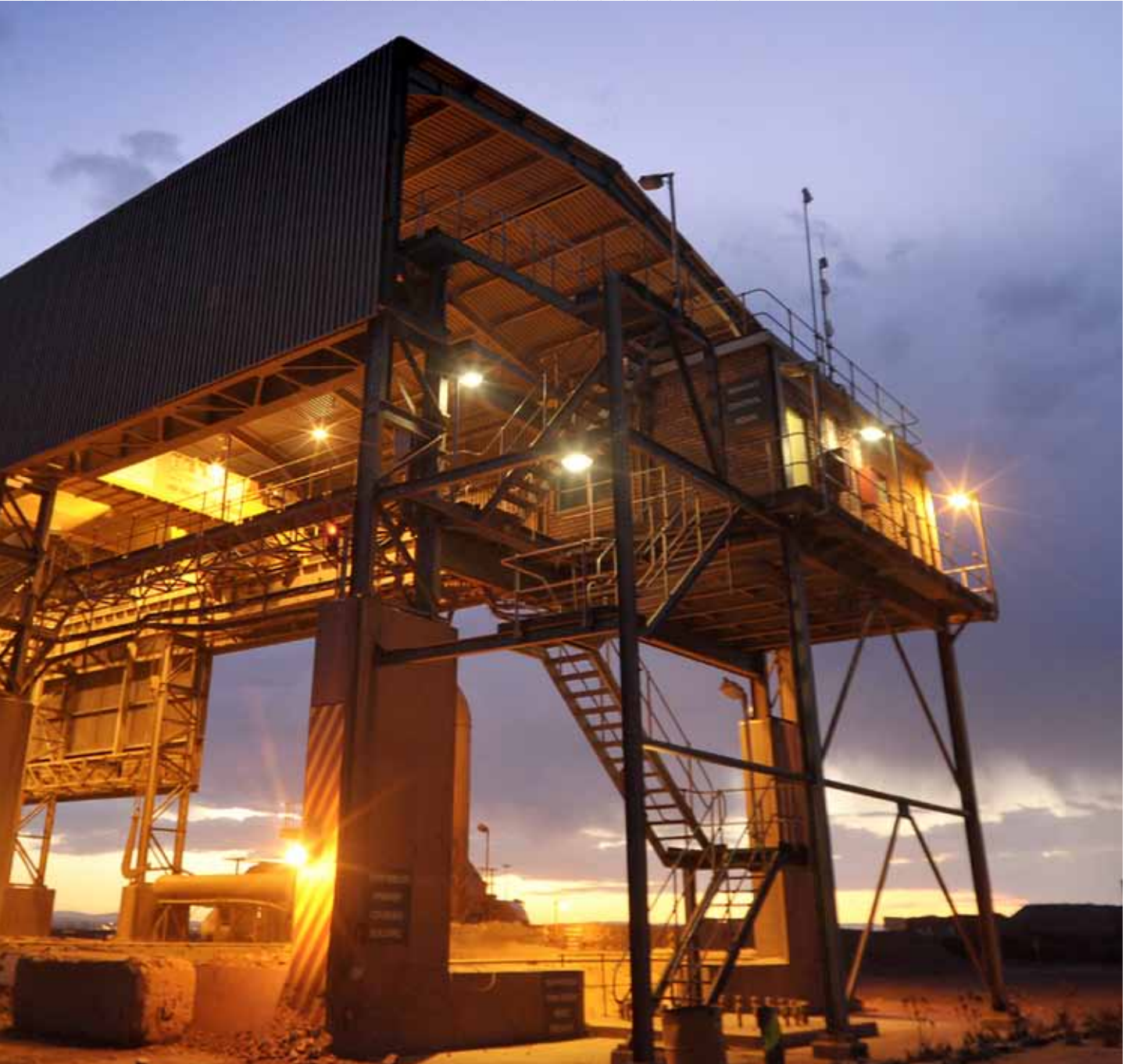
Primary crusher at Bruce.
