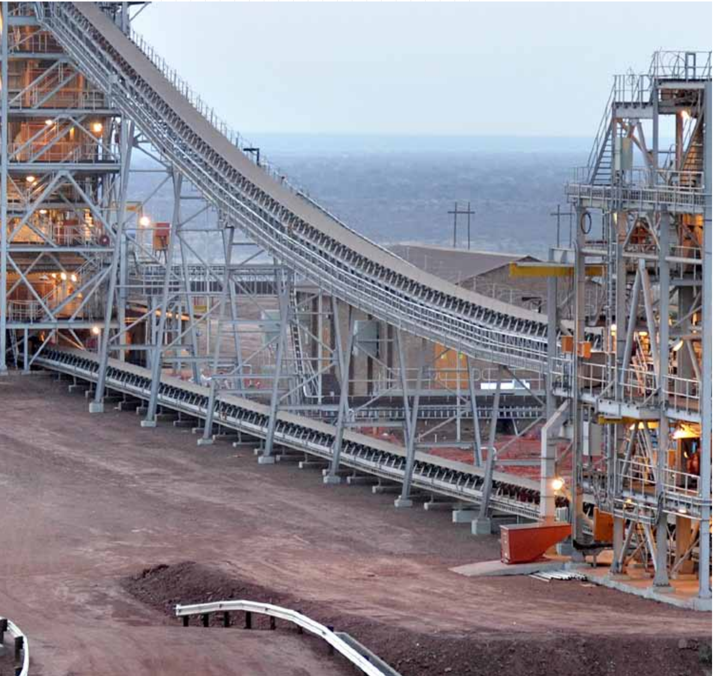
Construction of beneficiation plant on King (Khumani Iron Ore Mine).
