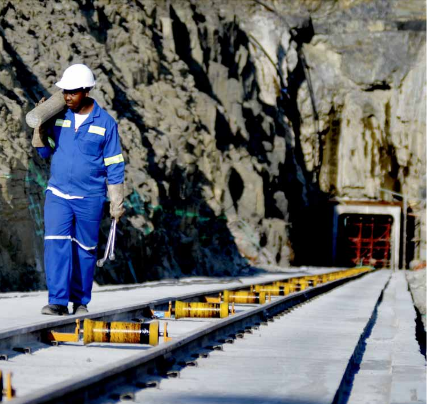
Zandspruit decline shaft at Rustenburg Minerals under construction.
