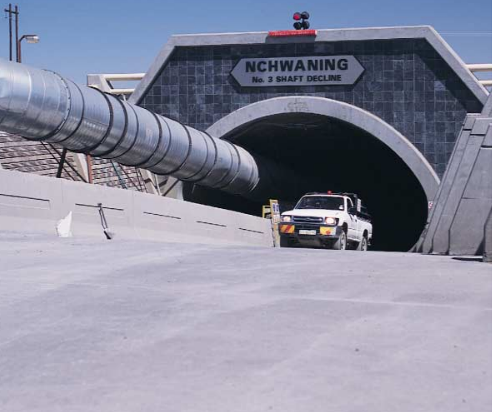
Entrance to the 2 200 metre long declined shaft being sunk as part of the N'chwanning 3 shaft complex scheduled for commissioning in 2003
