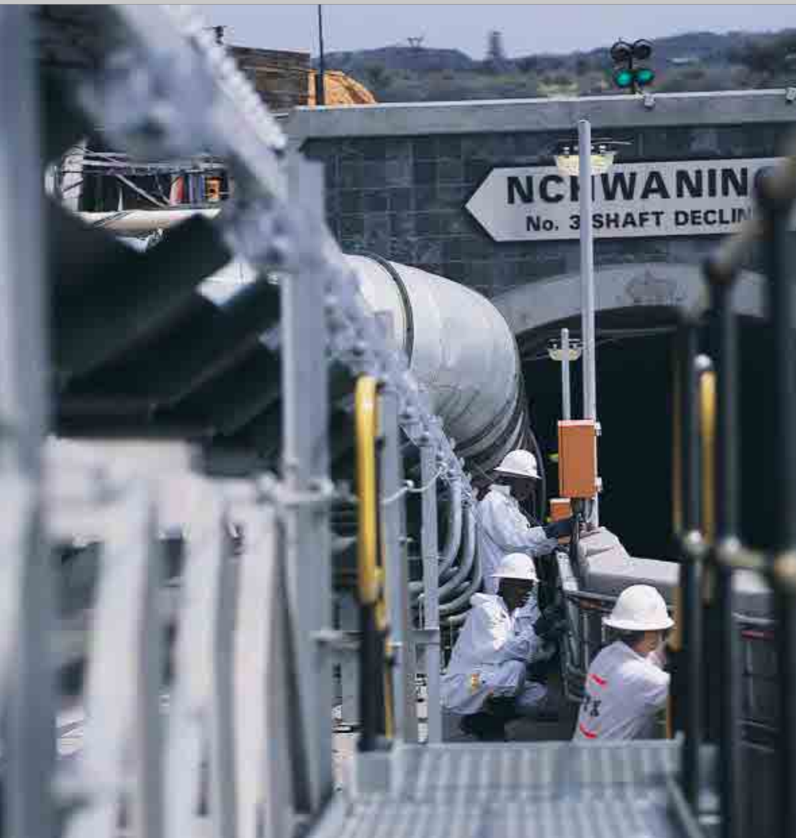
ENTRANCE TO NEW NCHWANING DECLINE SHAFT
